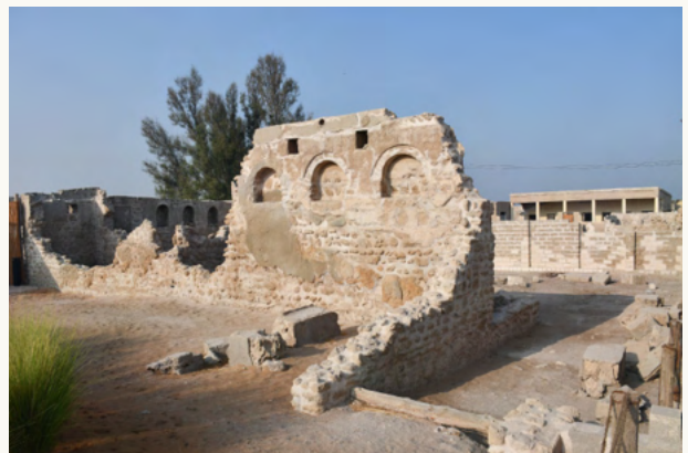
Figure 3: Conservation of a coral stone structure in Al Jazeera Al Hamra
