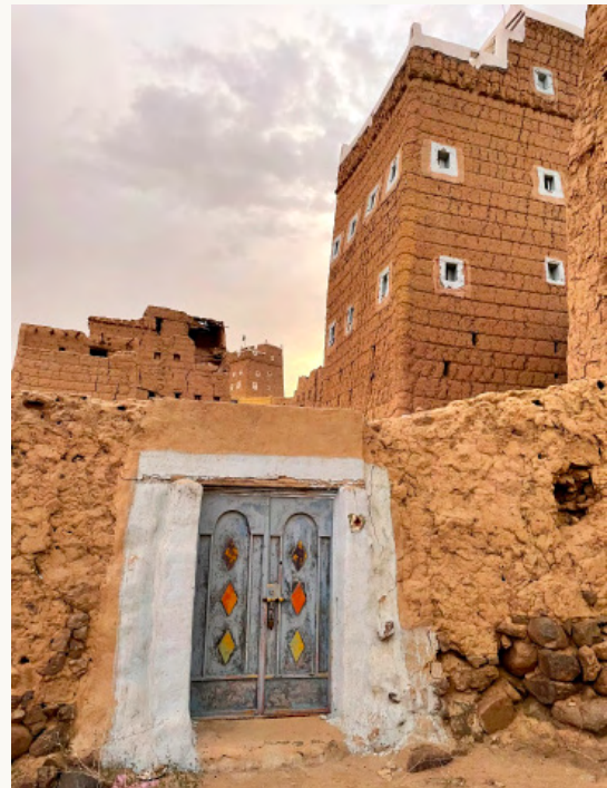
Fig 6 Decorative door installed at Zahran al Janub, Kingdom of Saudi Arabia. Photo by the author, May 2025.
