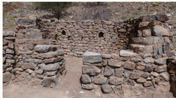
Figure 6 Restored late Islamic period house in Suhaila 2
