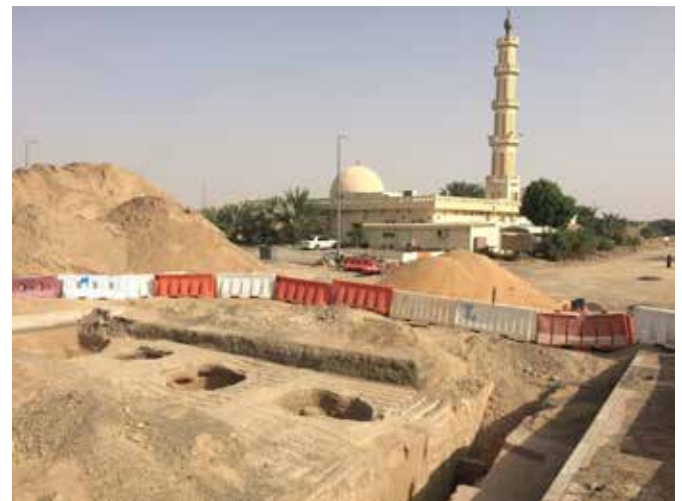
Closely spaced thuqāb in Falaj Al Mazmi
